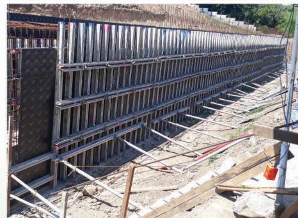
BATAAN BOX CULVERT
