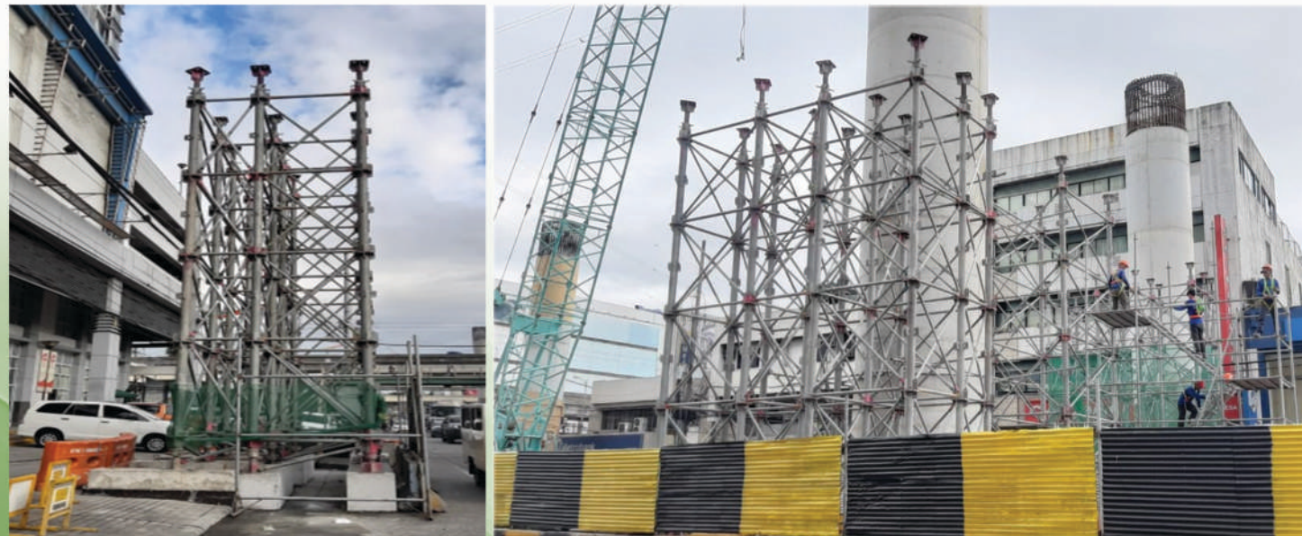
SAN JUAN VIADUCT SKYWAY STAGE 3B PROJECT
